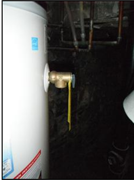
The relief valve should be diverted to the floor.
