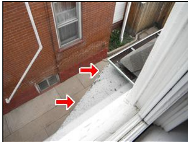
The small section of roof on the south side.
