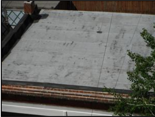
The garage roof.
