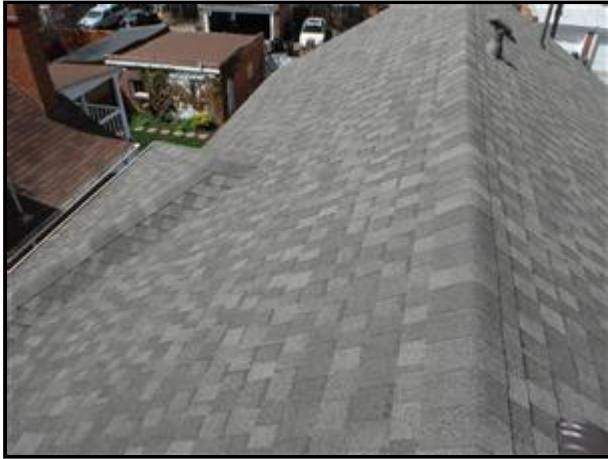
Overview of the south side of the roof.
