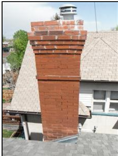
The west chimney.
