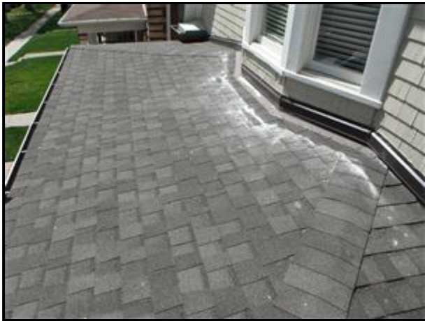
The roof on the front porch.
