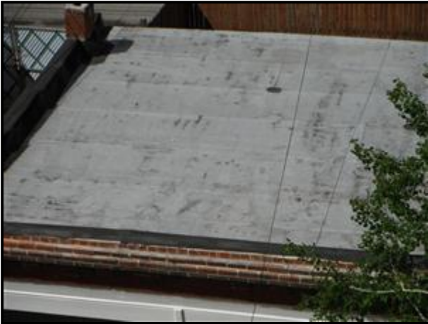
The garage roof.
