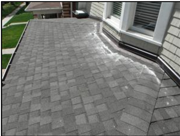
The roof on the front porch.
